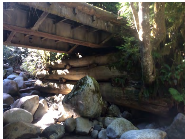
Left Bank Abutment when facing downstream
