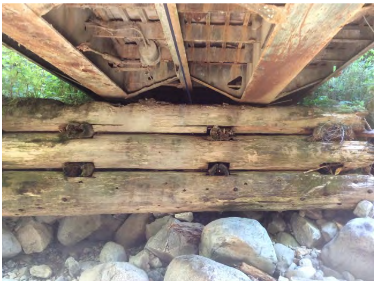
Right Bank Abutment when facing downstream
