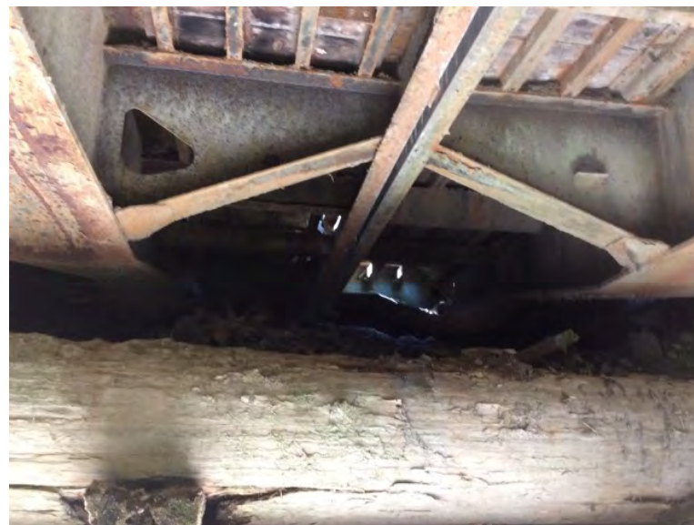
Left Bank Abutment when facing downstream
