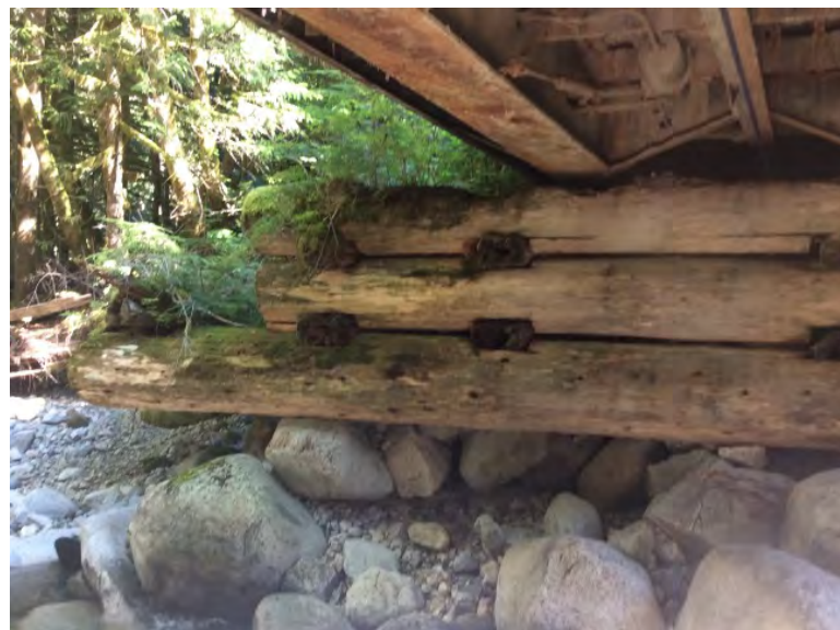
Right Bank Abutment when facing downstream
