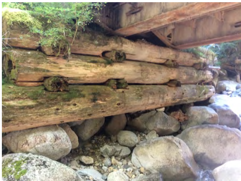
Right Bank Abutment when facing downstream
