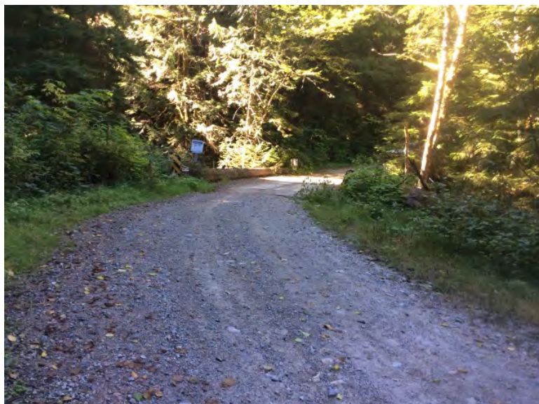
Approach from Right Bank when facing downstream
